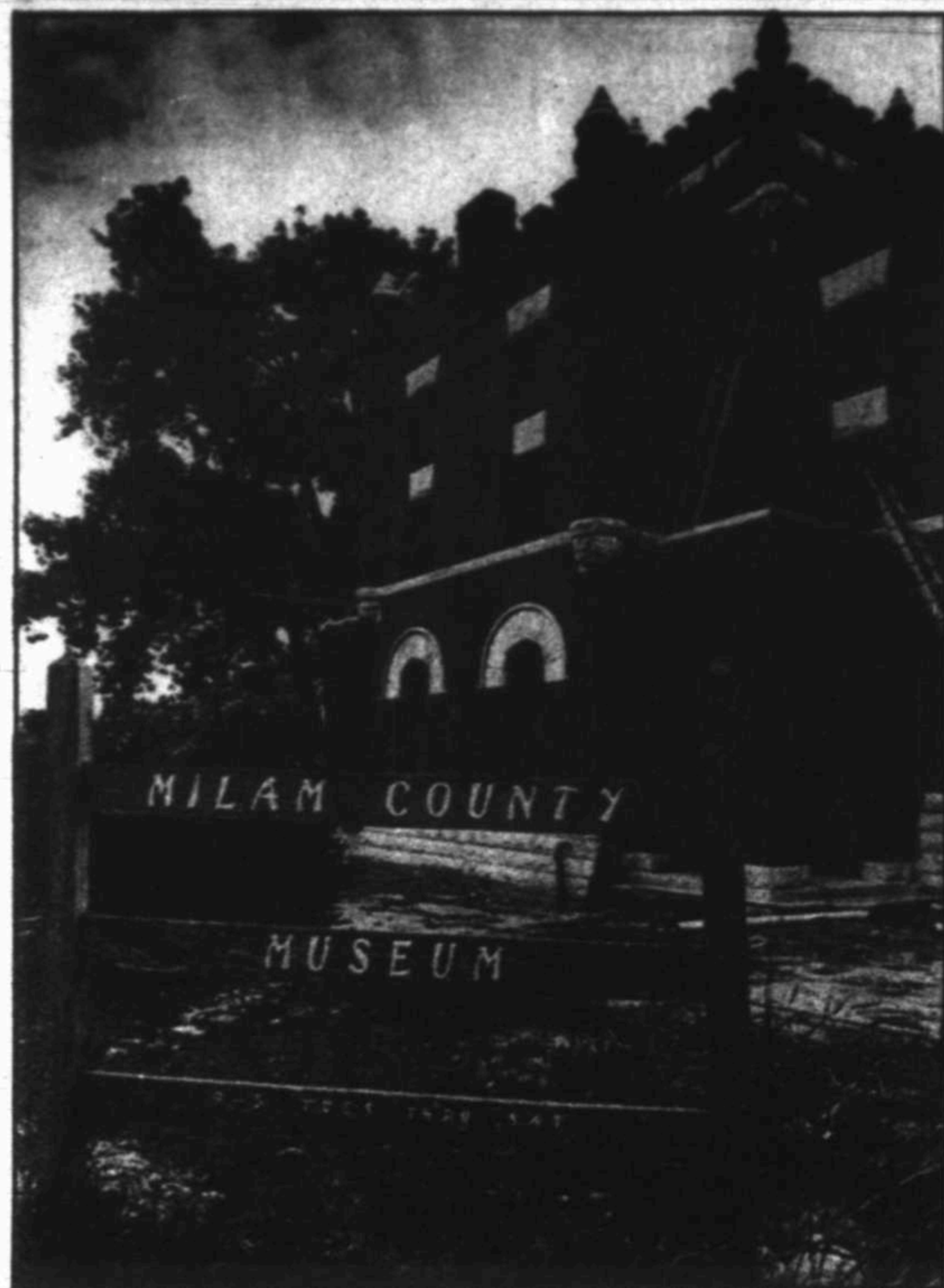
The former Milam County Jail, which served as a county museum from the mid-1970s until 1984, is being restored to its original appearance.
