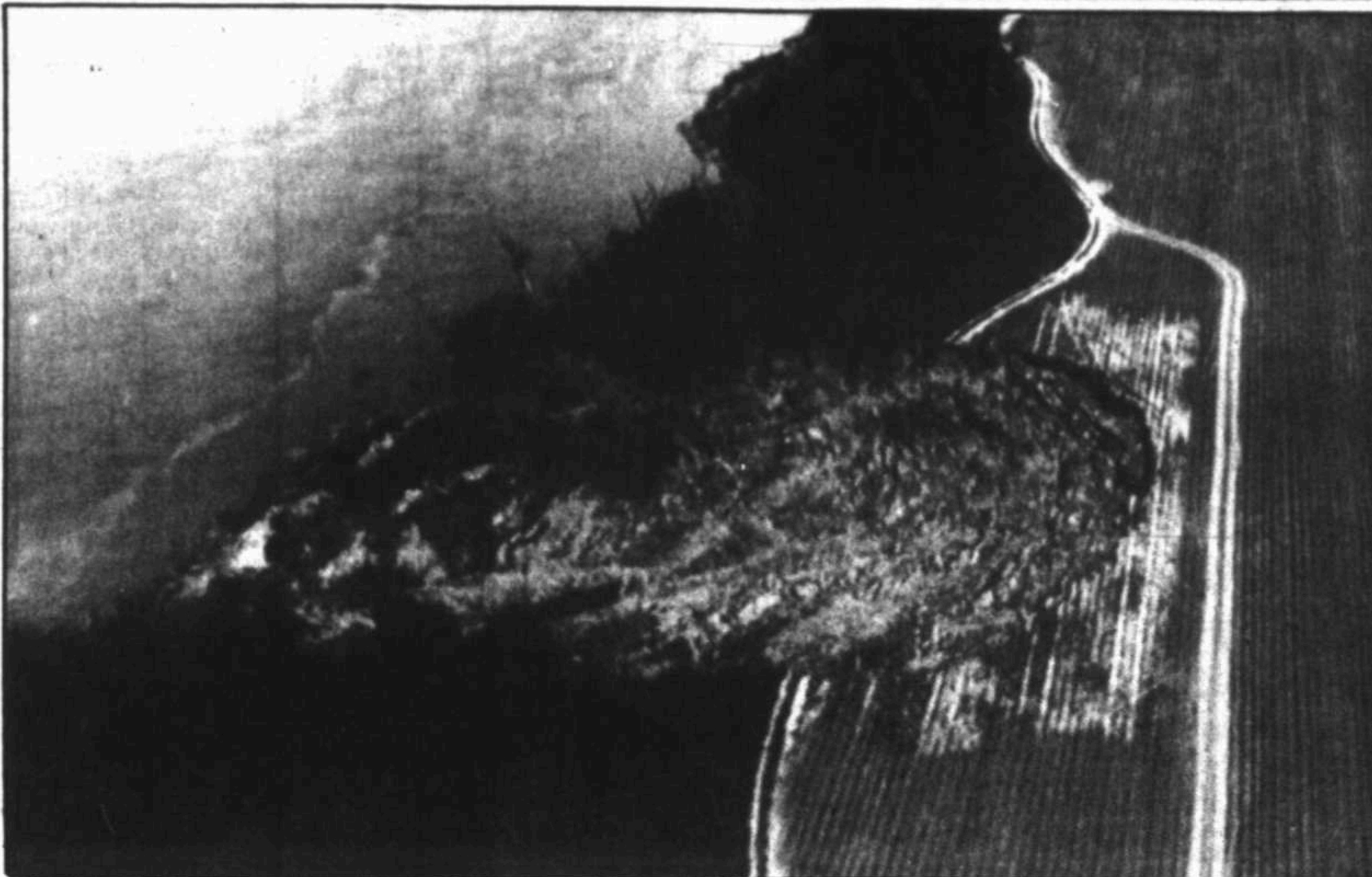
A riverside sinkhole covers about an acre of a soybean field near Helena, Ark. The hole appeared when the riverbank crumbled because of low water levels in the Mississippi River.
