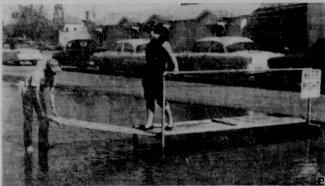
PORTABLE BRIDGE Midland, Texas' Ohio Street normally is a peaceful thoroughfare, but at those odd moments in Midland's life when it rains, it becomes flooded. So, City traffic engineer Jack Keese decided to do something about it. He invented the portable pedestrian drawbridge, which can be extended to fit the size of the puddle. Above, city employee S. J. Cooley extends the bridge for Margie Louise Robertson during its tryout. The bridge was a success as 36 grateful pedestrians scampered across the bridge in a ten minute period.—L.P. Photo.
