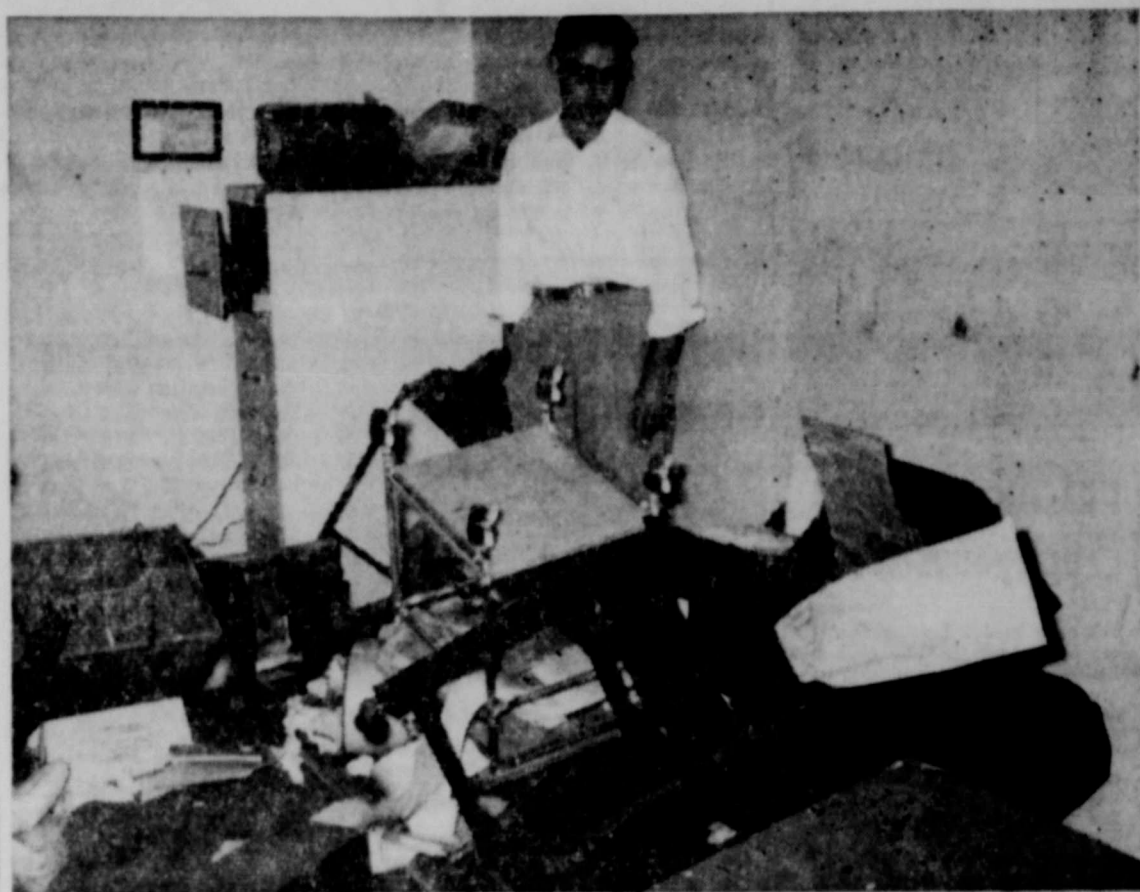
EXPLOSION DAMAGE—Max McLarty of the Community Public Service views the damage suffered in an explosion at the company warehouse Friday morning. The blast, believed to have been caused by an accumulation of gas under the floor and in the walls, damaged the equipment of the billing office. McLarty escaped serious injury, but was blown through the door by the blast.
