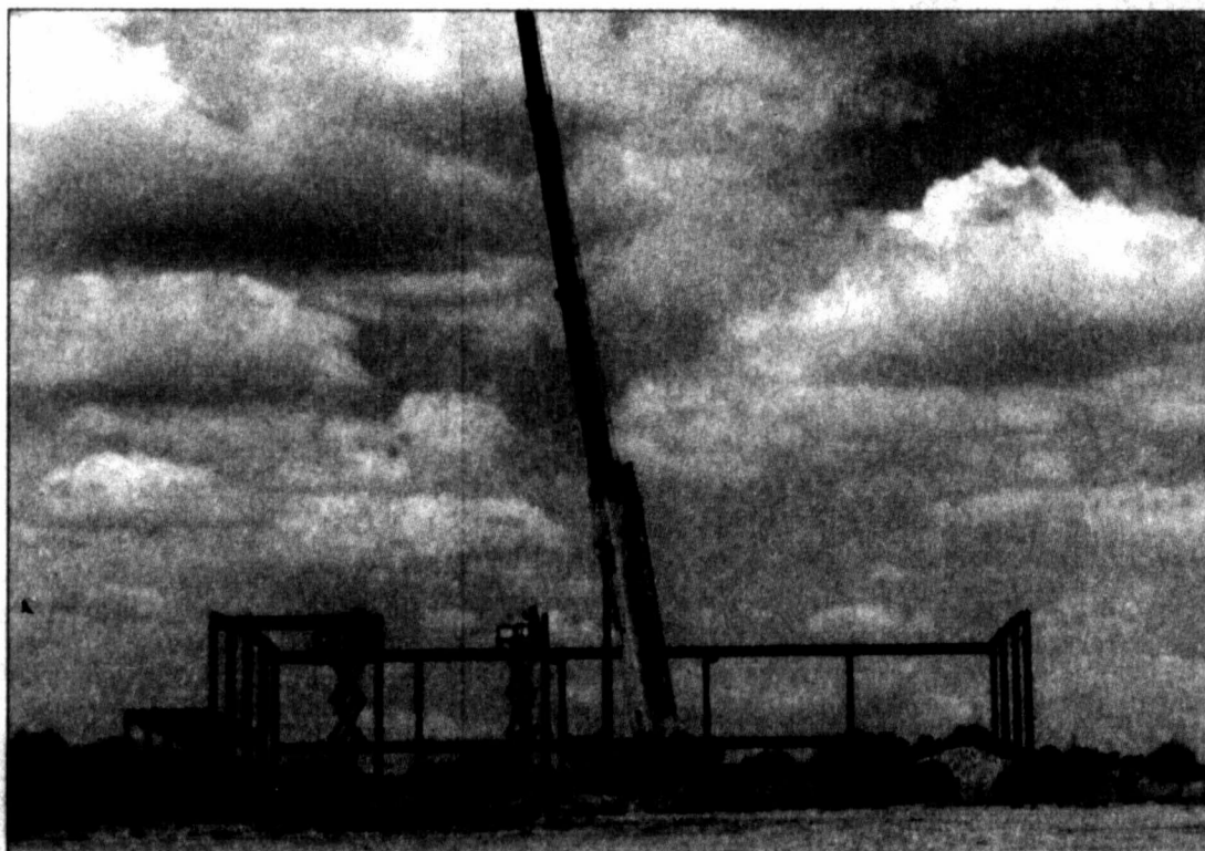
GOING UP - The first steel beams were erected early this week at the site of the new Colorado ISD K-8 campus. Construction crews were working diligently to put up the steel that was delivered to the site last week.
