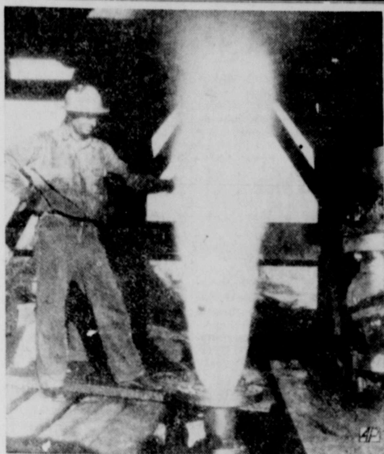
JUST ANOTHER JOB—John Jobe, expert oil well fighter from Houston, stands at the base of a wild gas well at Tyler. The dangerous job of capping the well is just another job to him, Jobe said. Early efforts to cap the well failed because of the strong pressure. The spray of gas caused officials to evacuate the surrounding area, hoping to avoid a serious fire. (AP Photo)
