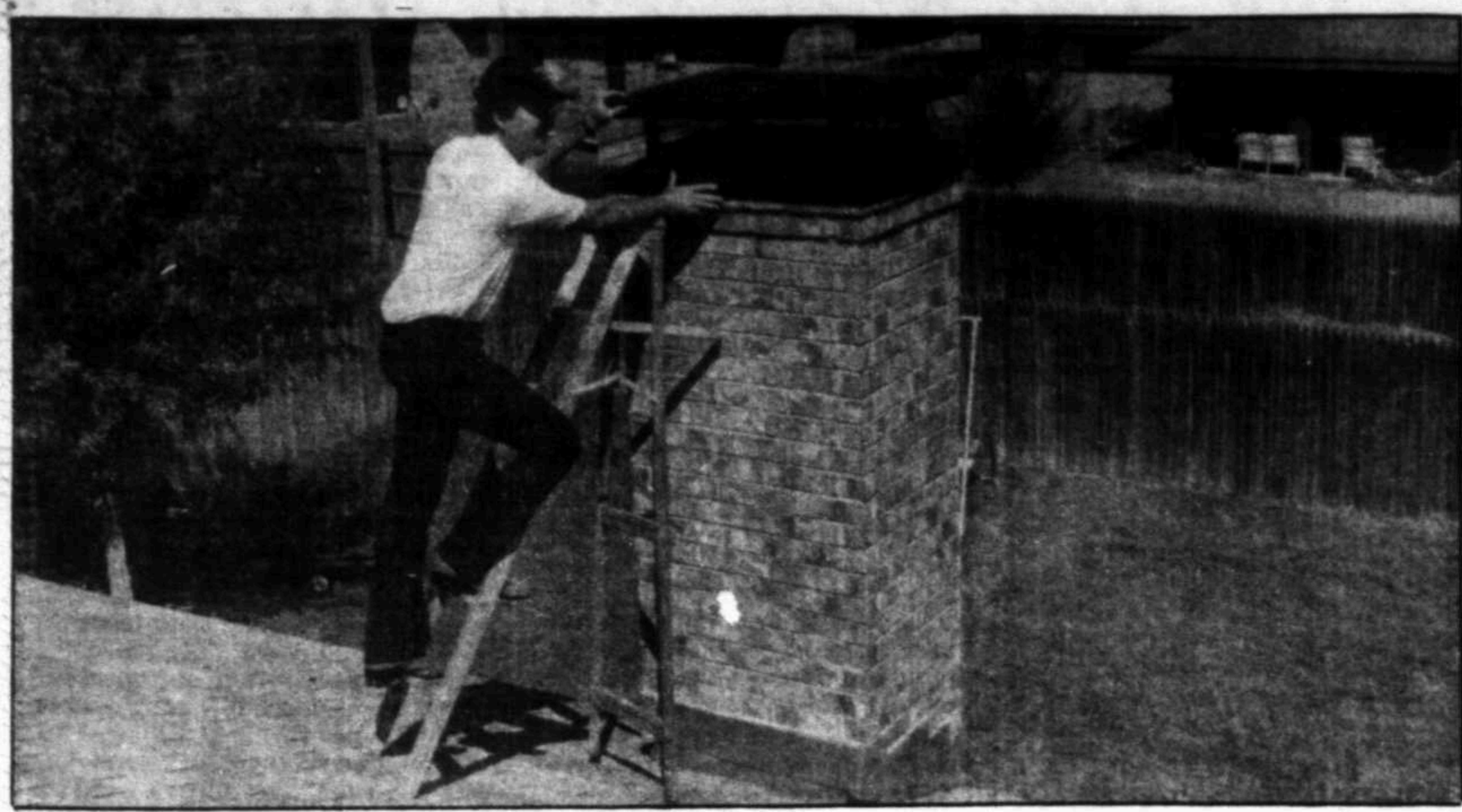
All Seasons Chimney Service installs custom caps, measured and designed to fit each individual fireplace. Ernest Meyer, owner of All Seasons Chimney Service, is shown installing a cap after a chimney cleaning. For a free estimate call 697-7585 between 8 a.m. and 5:30 p.m.
