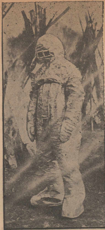
FLAMEPROOF FIREMAN— Walking through flames unsinged is this German fireman seen above. He is demonstrating protective qualities of a flexible, aluminum fireproof suit at an exhibition held in Essen, Germany.
