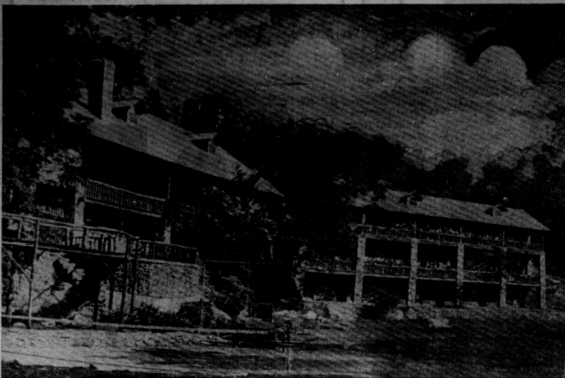
ALL OF THE FACILITIES of the famous Heart o' the Hills Inn near Kerrville are converted to camp activities every June and July. Shown above is the main air-conditioned
