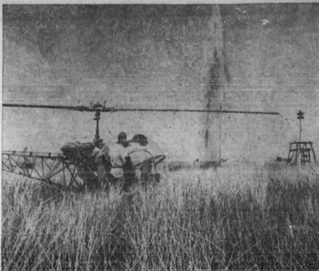
OIL WILDCATting GOES SCIENTIFIC — In marshy country special equipment must be used to carry on the endless hunt for oil clues. Here a seismic crew flown in by helicopter fires a dynamite shot to "sound out" possible oil-bearing formations located far below the earth's surface.
