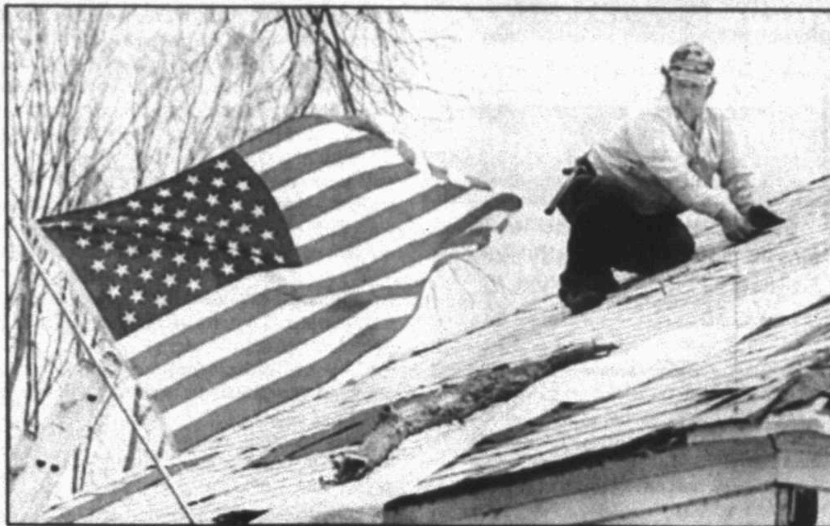
Pedro Hernandez patches a tornado damaged roof on the west side of Fort Worth, Thursday. A tornado swept through the neighborhood Tuesday evening before hitting the downtown area.
