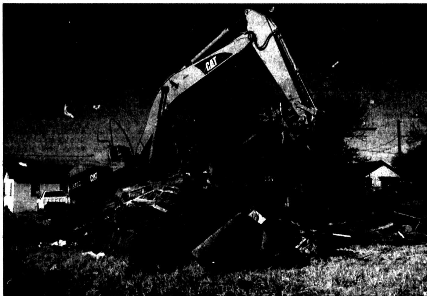
A private contractor tears down an abandoned building during Saturday's Coahoma Trash Off, which targeted nearly a half-dozen dilapidated structures in the city for demolition. The Trash Off was part of the Rural Community College Initiative (RCCI) effort to revitalize the community.
