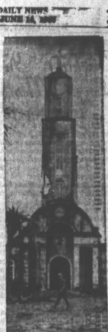
CASUALTY OF WAR—a gutted church steeple poles skyward in a Vietnamese jungle clearing. It has been pressed into service by both the Viet Cong, as a sniper position, and U.S. Marines, who used it as an observation post during a field operation in Quang Ngai Province.
