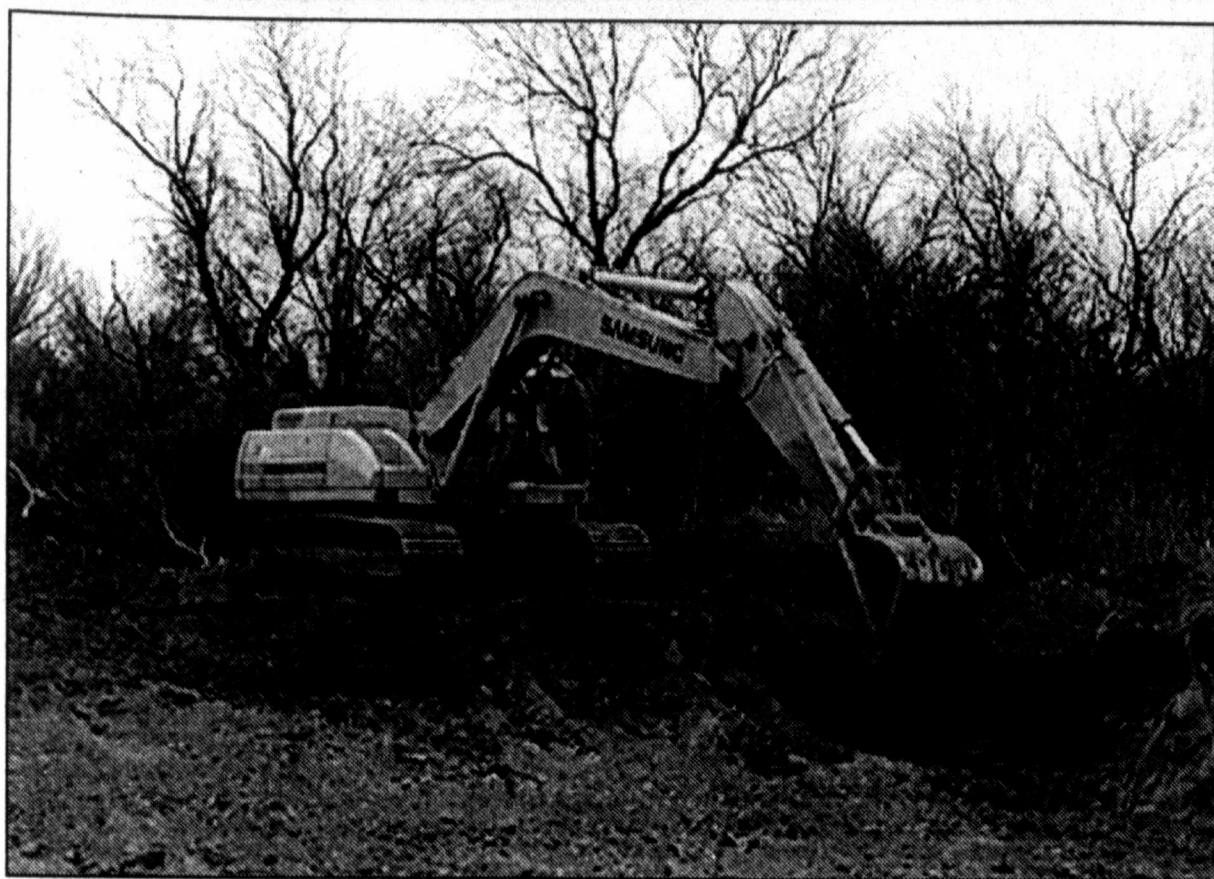
NARROWING THE COLORADO RIVER is necessary before a water line can be laid under it late this week. Marcial Ramirez of Midland was working on the north side of the river in southwestern Colorado City Tuesday.
