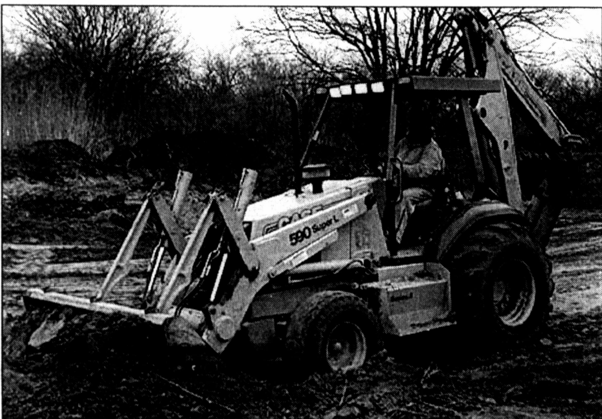
PREPARATORY WORK to laying the new city water line under the Colorado River south of Lafayette Street was underway Tuesday afternoon with this Thane Ditching Co. machine. Thane, of Odessa, is one of three companies working on the $3.5 million project.
