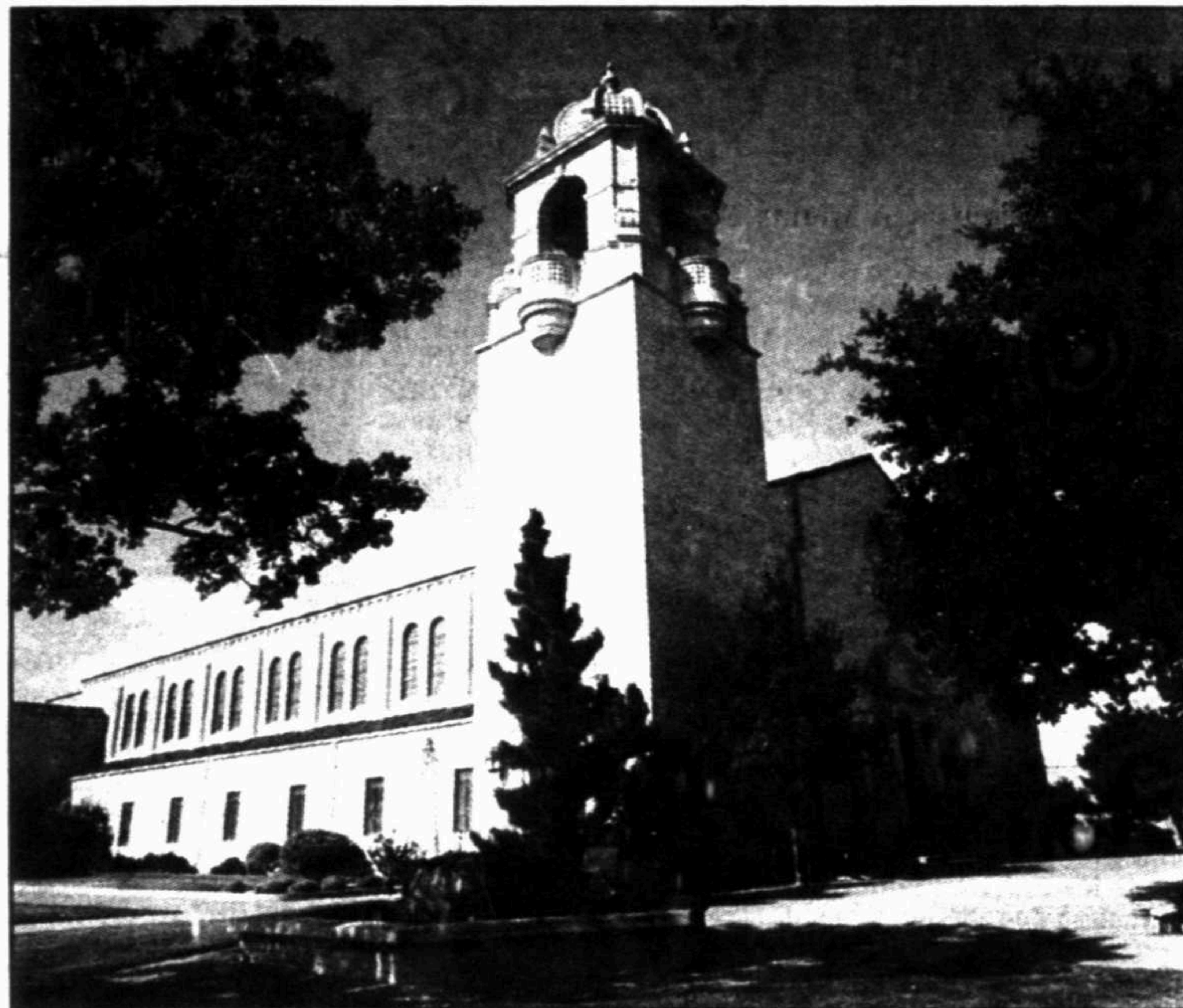
Maintenance at First Baptist requires 10 full-time employees, who work under the supervision of Randy Matthews.
