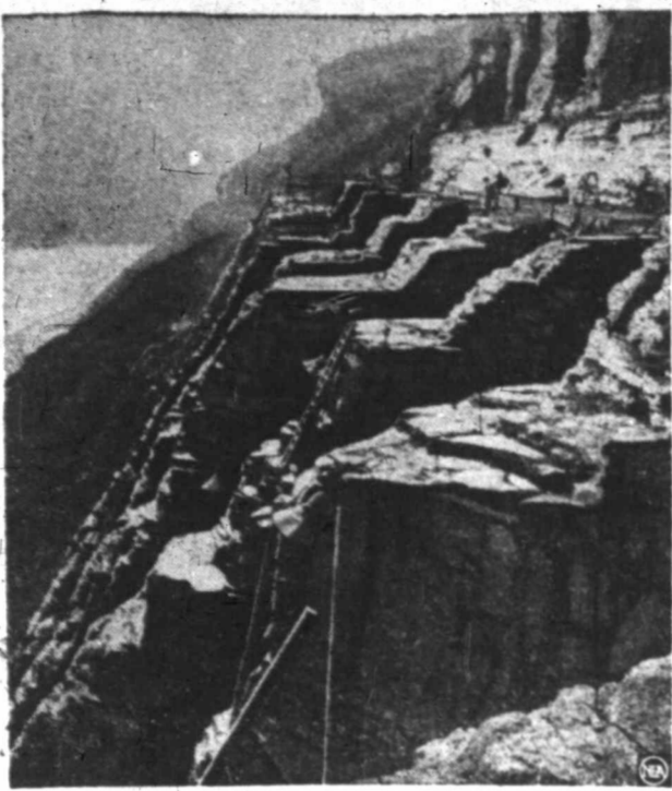
Power penstocks: This is part of the rock-blasting being done on the shore of the Niagara River (seen faintly at left) for the seven penstocks that will bring water from Niagara Falls to a new generating station to create 700,000 horsepower.
