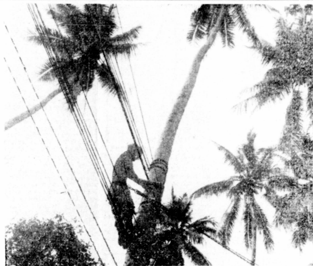
THIS YANK IS UP A TREE—Sergeant Nelson Waterbury, of Ypsilanti, Mich., may be up a tree on New Guinea Island in the South Pacific, but it's all for a good purpose as he checks the lines of communication strung in palm trees serving as telephone poles.
