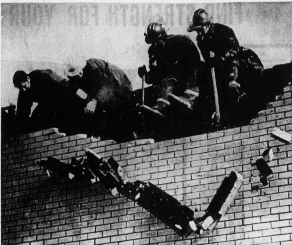
DOWN IT GOES — Lubbock firemen knock down part of a wall at the Village Inn on Brownfield Highway in search of "hot spots" left after a fire early this morning. The blaze was concentrated in the roof and attic. (Staff Photo)
