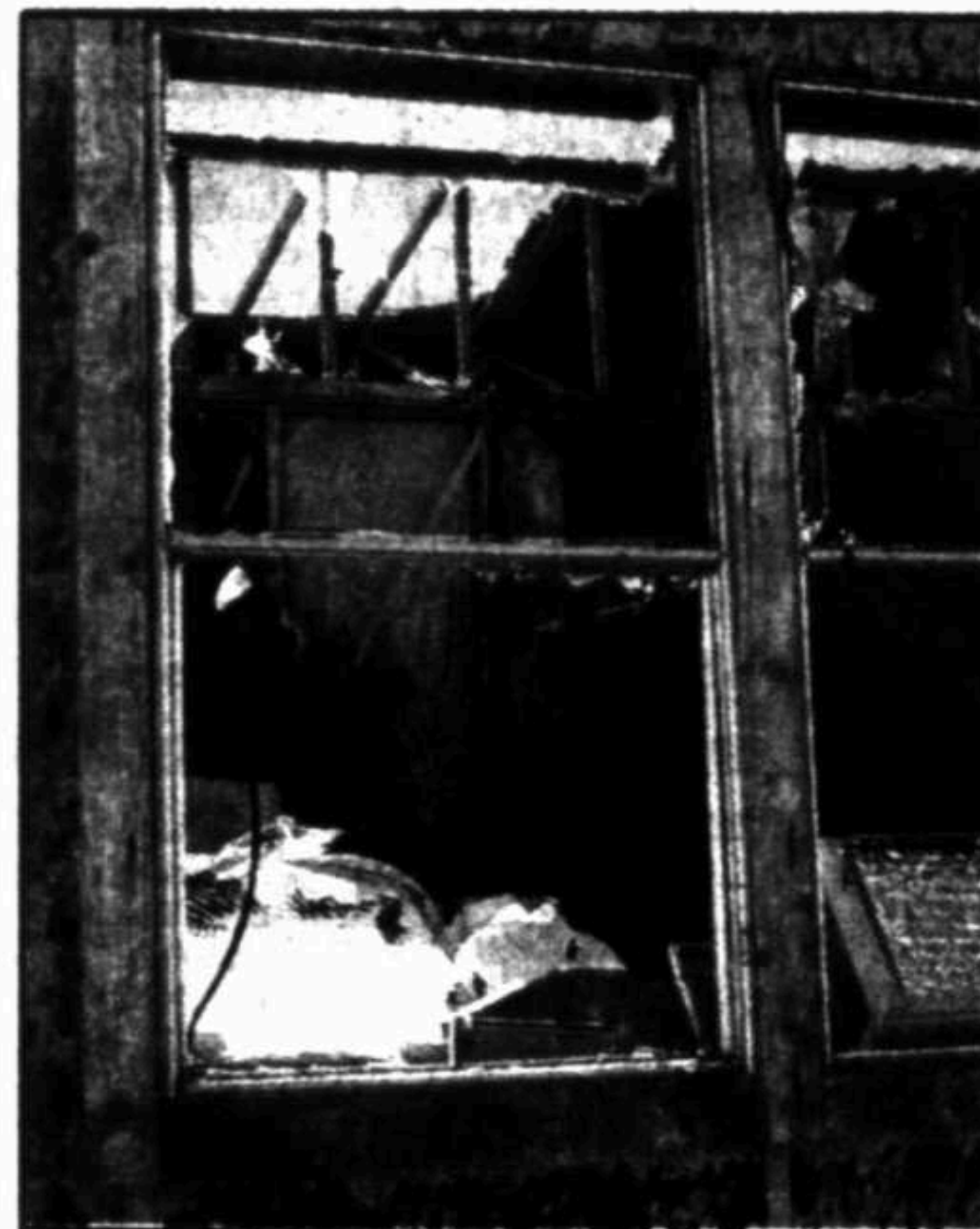
Tim Fischer/Reporter-Telegram This home was among those damaged by hail and high winds Tuesday night.
