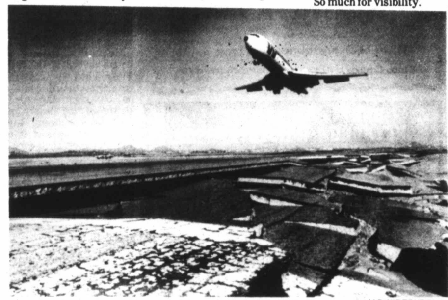
ROUGH RUNWAY — A commercial airliner takes off from Phoenix Sky Harbor International Airport Wednesday despite crumbled hunks of concrete at end of main runway. Repairs to runway and taxiway, caused by last week's flooding of Salt River, are estimated to cost about $4 million.
