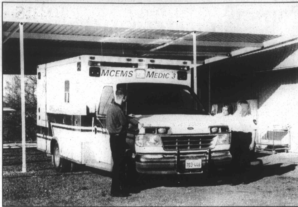
MITCHELL COUNTY EMS Director Jason Cooper talks shop with emergency medical technicians Ava Ramirez and Kristi Cox at the ambulance bays that are under construction at the company's new headquarters on Westpoint Street.
