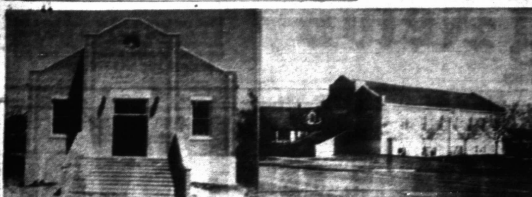
NEW SANCTUARY—The First Christian Church, Miami, is shown from the front in left view. Right shows the sanctuary from the side. It is a monument to years of effort. (News Engraving)
