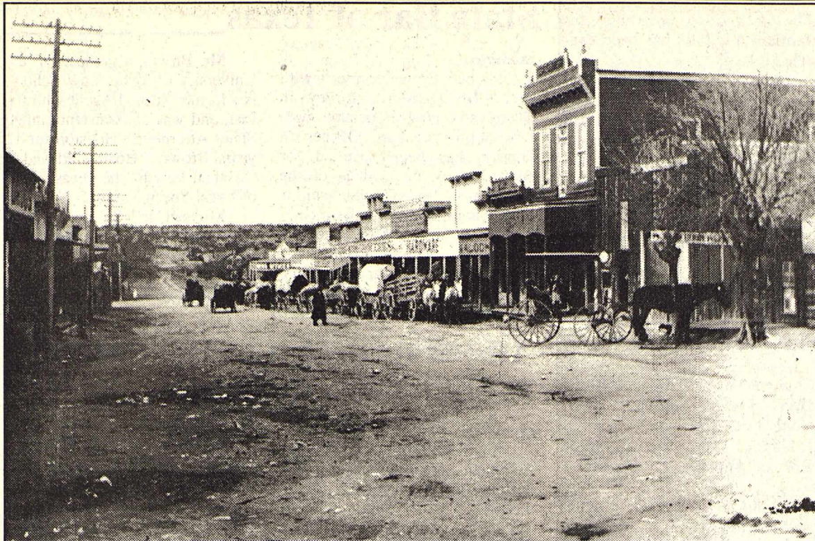
Koenig/Craddock/Medical Arts Bldg. is the 2 story building on right in this approx. 1920's photo.
