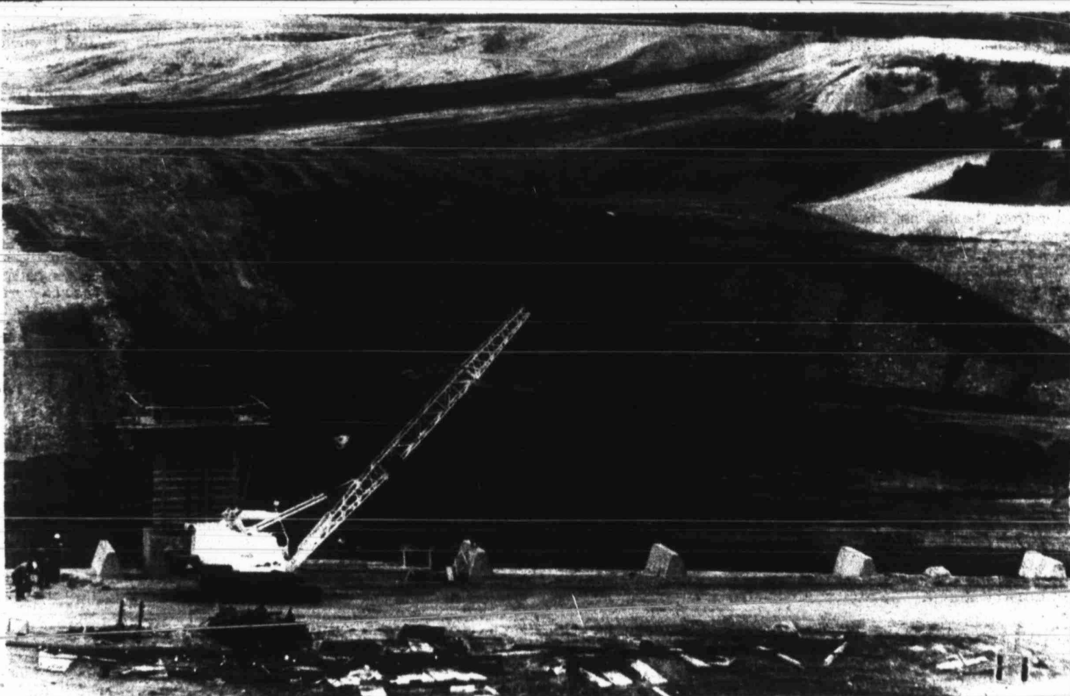
A crane works in what will be one of the low points in the Red Draw reservoir.
