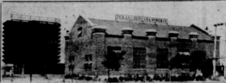
PERRYTON CENTRAL POWER PLANT
