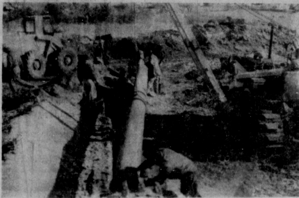
Connecting Water Line
