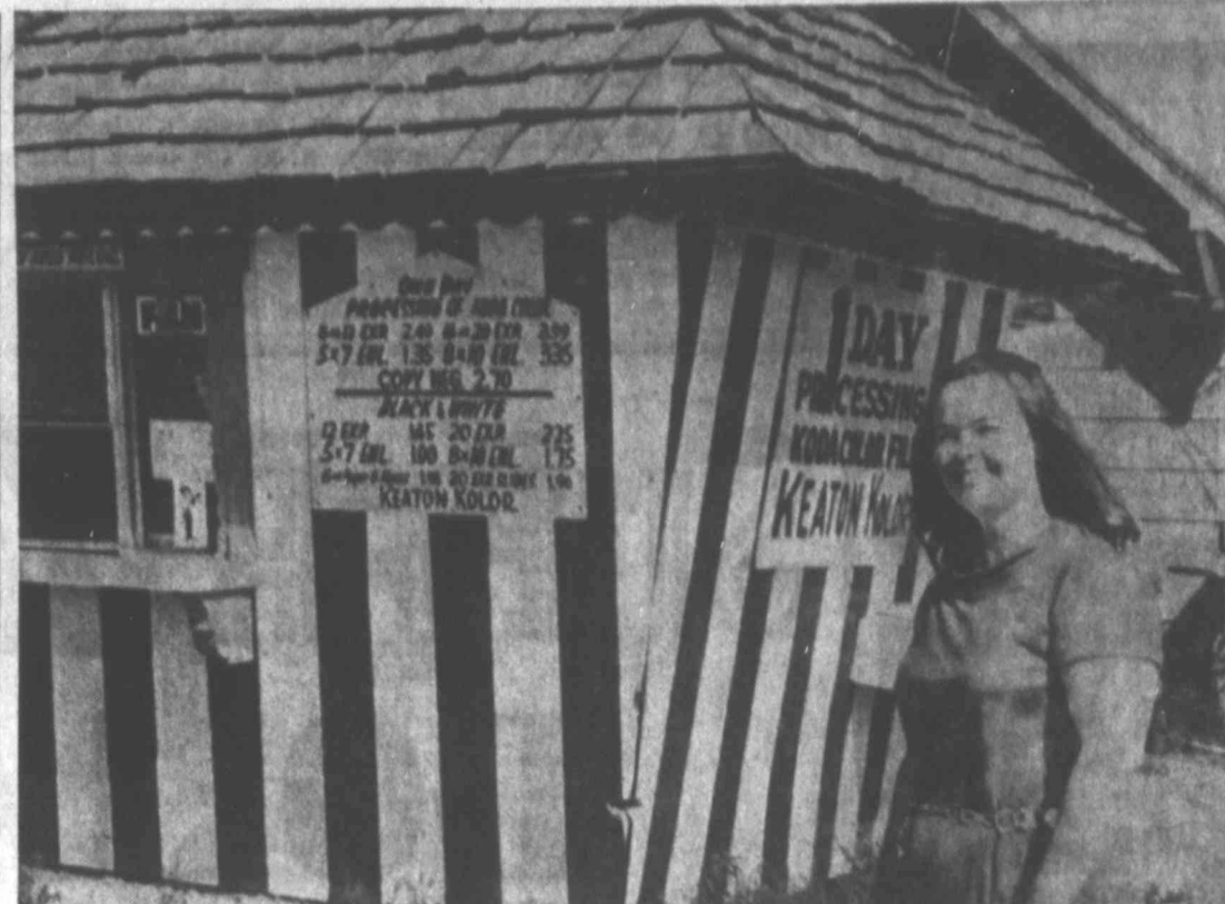
KEATON KOLOR PHOTO PROCESSING ... the candy-striped building on Gregg
