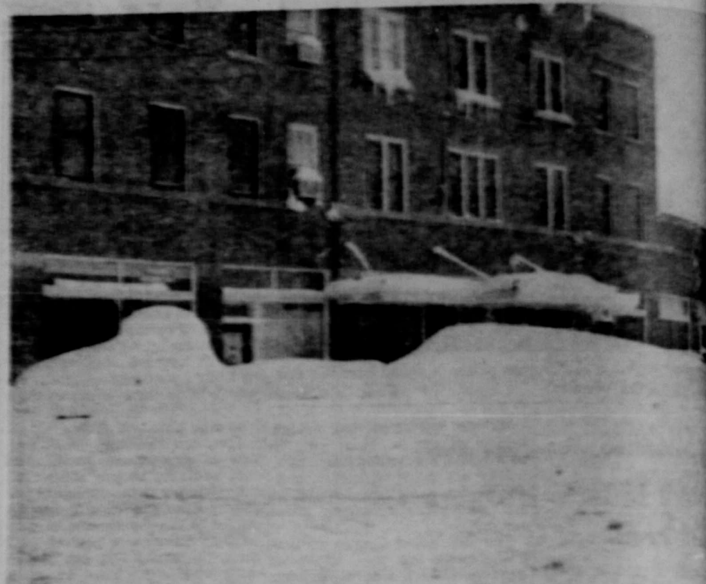
SNOWBOUND —Travelers at the Hotel Perryton could see practically nothing but this outside the main entrance which covered up the entire half block of automobiles.
