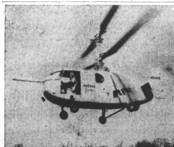
BIGGEST WHIRLBIRD —Jim Ryan, of Port Jefferson, L. I., takes largest privately built helicopter in America up for its test flight. The coaxial rotor helicopter was manufactured by Cyrodene Company, and is being tested under military contract. It can carry six to seven passengers, or crew of two and three litter patients.
