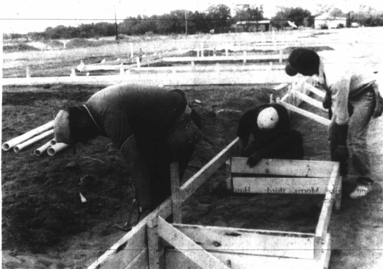
PPI HOMES UNDERWAY —Foundation slabs are poured for five new homes. The housing for low income families, located north of the swimming pool, is a People for Progress, Inc. project. The long awaited construction on the homes began last week and is expected to be completed by the first of next year.
