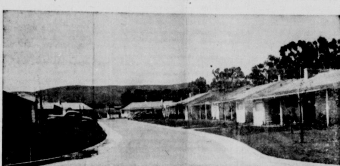
A very satisfactory type of curb and gutter has been installed in this California subdivision. At street corners the curb is vertical but along the interior lots it is sloping. This feature permits driveways to be located anywhere without cutting curbs or making special aprons. Federal Housing Administration land planning officials describe this as a practical treatment which could be copied in many low-cost subdivisions.
