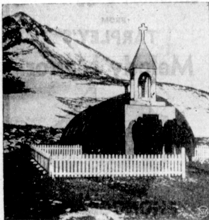
LITTLE CHURCH AROUND THE POLE —This tiny quonset hut chapel at Hut Point, McMurdo Sound, Antarctica, will be crowded at Christmas. Erected for personnel of the Navy's "Operation Deep Freeze" around the South Pole, it has had religious services every Sunday.
