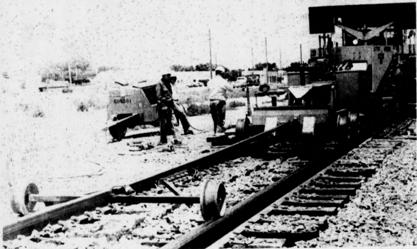
Working on the railroad
