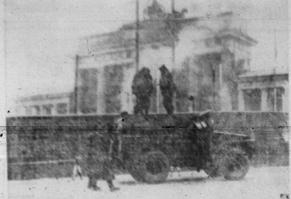
MORE BARRIERS FOR BERLIN —British soldiers peak over top of the new 12-foot barrier, hence erected by the Communists along the Berlin east-west border near Brandenburg Gate in the background. The screen was put up to shield workers laboring under armed Red guards as they erected reinforced concrete barriers and tank traps along the border. Two West Berlin policemen on border duty walk past the British armored car. (AP Wirephoto via radio from Berlin)
