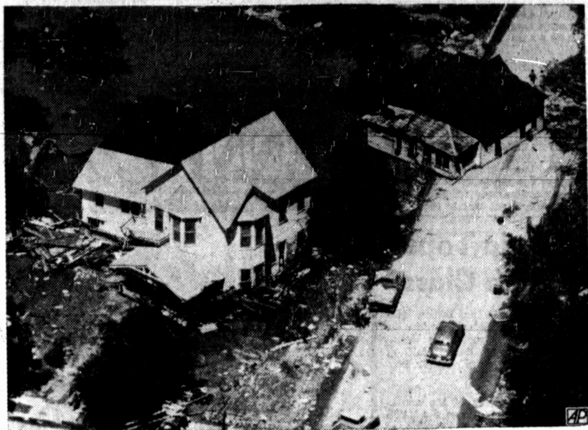
Ripped Off Foundations
