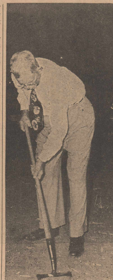
L. D. BARTLETT . . . ... breaking ground for new church
