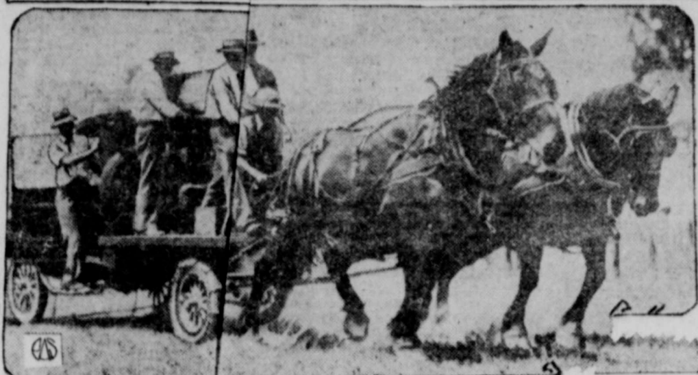
"Bill" and "Colonel," the team belonging to George Wilcox, of Greenville, Ohio, pulling against a motor truck, at the Jay Court fair, made a record of 3,550 pound drawbar pull, equal to hauling 46,102 pounds on a wagon or
