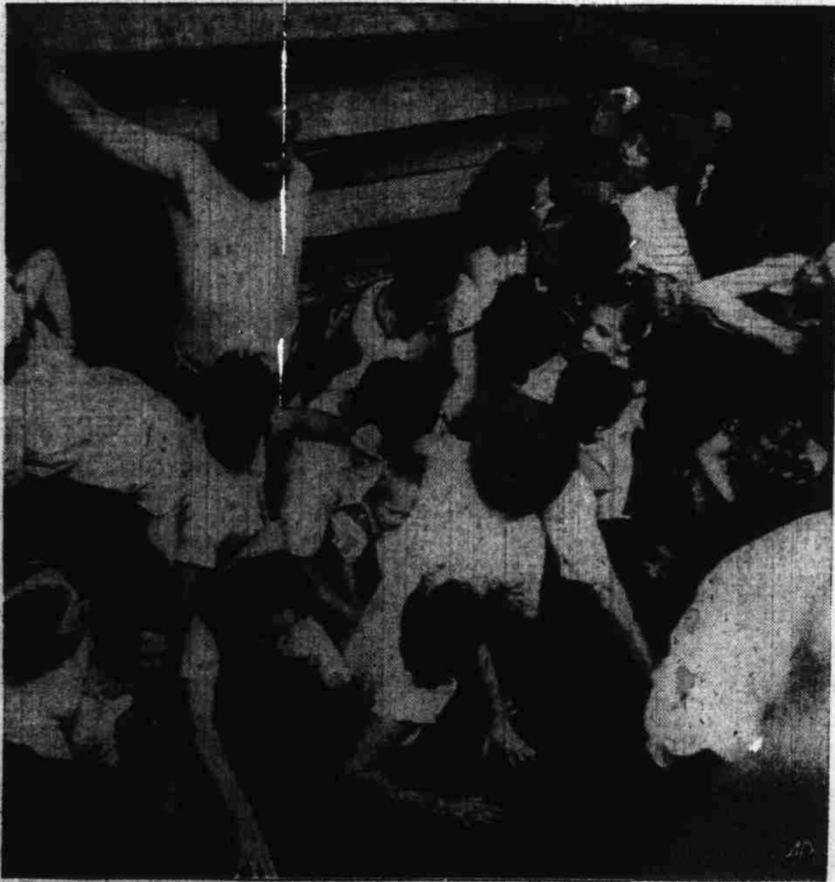
SCRAMBLE AS PIER STEPS COLLAPSE—Part of the 40 persons who fell 17 feet to the bottom of the Galveston Bay, seawall when entrance steps to a pier collapsed are shown just after they fell. The list of injured totaled more than 37. Accident occurred as Galveston held Splash Day Celebration opening its beach. (AP Wirephoto).
