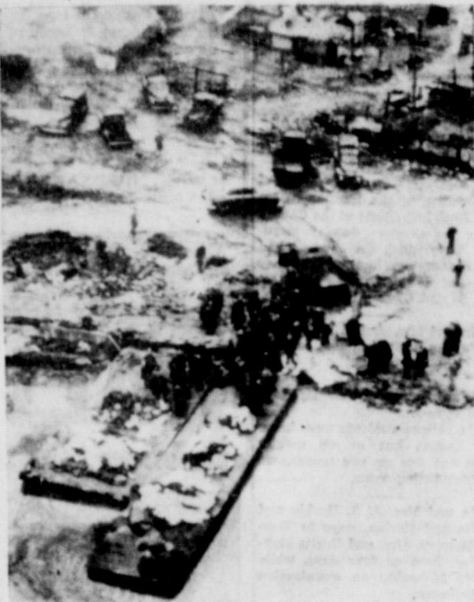
SANDBAGS FOR LEVEE —Weary workers, toiling in a sea of mud, unload sandbags from Army barges brought in to bolster levee at East Omaha, Neb. Army Engineers say that pumps are keeping up with seepage at critical points. (NEA Telephoto).
