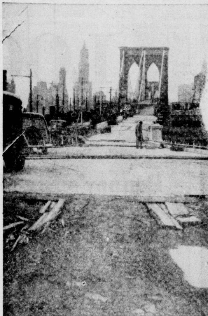
ALMOST FINISHED—Work on the new Brooklyn and Manhattan approaches to the Brooklyn Bridge spanning the East River is about finished. The Department of Public Works began a "face-lifting" in 1950 but steel shortages and bad weather delayed completion of the project. This photo showing the resurfacing was made from the Manhattan side of the river looking east.
