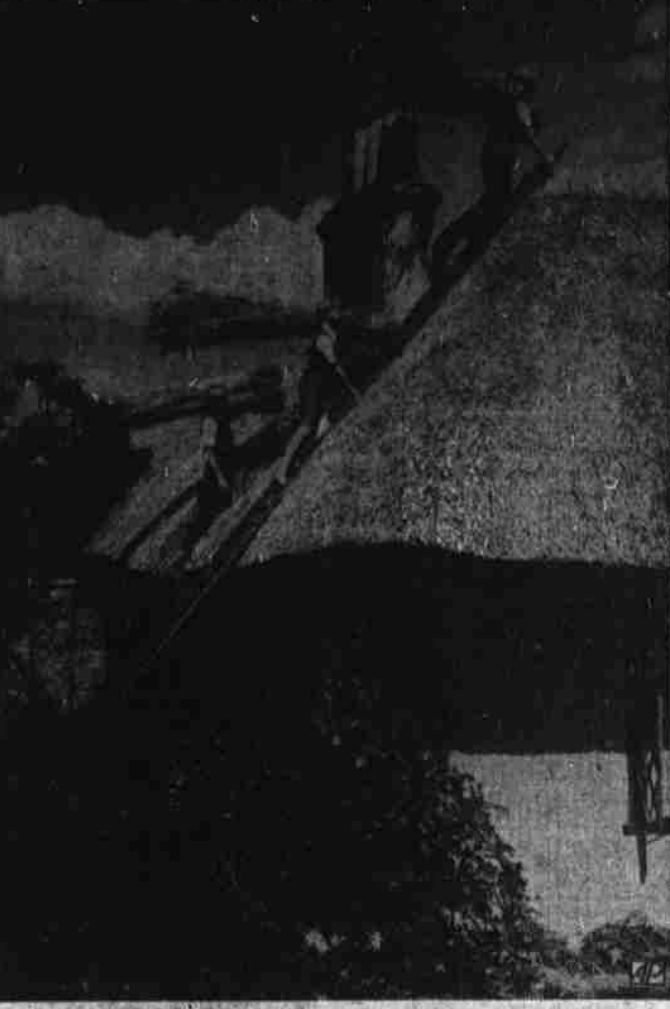
ON THIS ROOFING JOB bundles of reeds were used for this is "The Hermitage" at Hanwell, one of the few thatched houses in vicinity of London. Reeds are used for rethatching house which was built by the Rev. G. H. Glasco.
