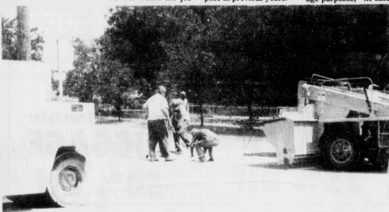
ROAD CONSTRUCTION-Price Construction Company is currently seal coating Elm Street. The road construction began early this week.
