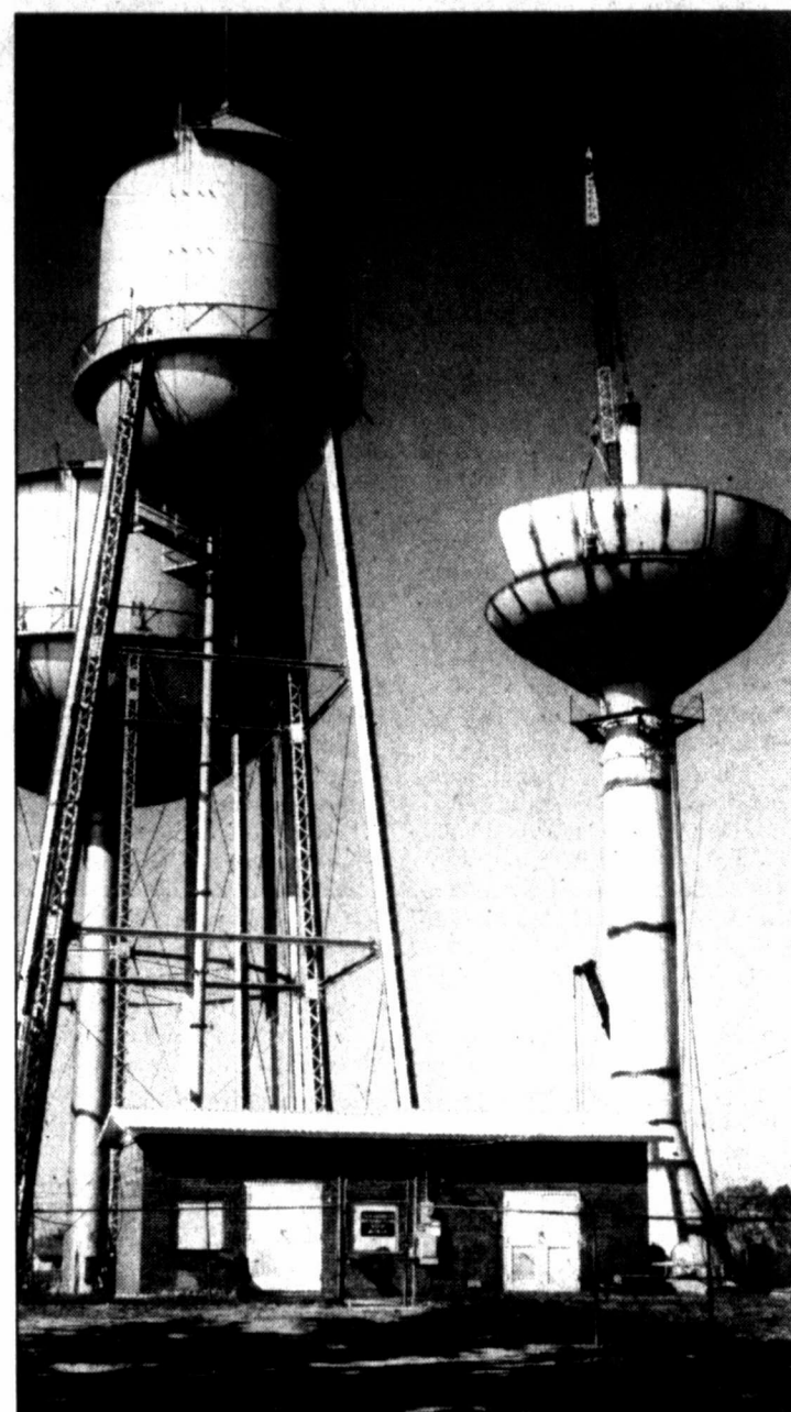
BUILDING INTO THE SKY – The construction of the city's new water tower is progressing well and ahead of schedule. Soon the city will decide on a logo and paint scheme, according to City Manager Fabio Angell. When completed and in use, the two older water towers will be torn down.
