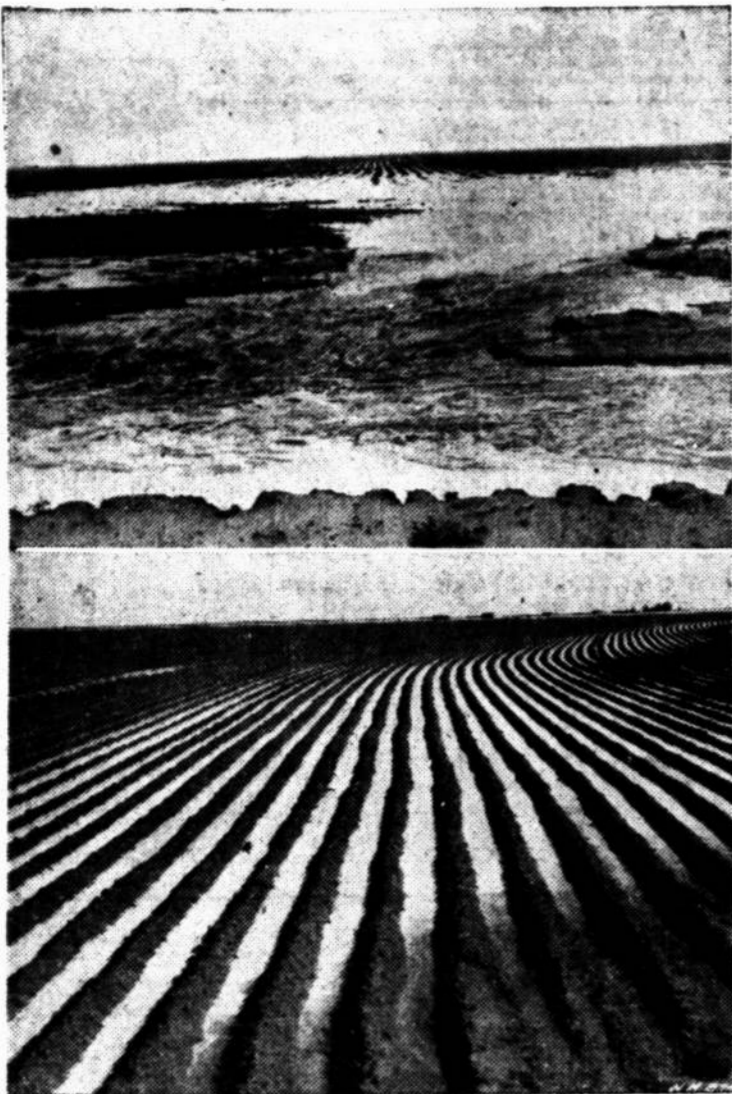
Proper control of water is necessary to prevent soil erosion and to insure successful crops, the Soil Conservation Service says. Straight rows up and down slopes (shown at top) serve as miniature drainage ditches which allow water to flow off land where it falls. This rushing water is taking a heavy load of valuable topsoil and is being lost for use in growing crops, to say nothing of adding to flood danger downstream. Contour rows (shown at bottom), strengthened by terraces where necessary, hold practically all the water on the land. This insures even crop stands, better yields, prevents soil losses and gullying and tends to check flood damage.
