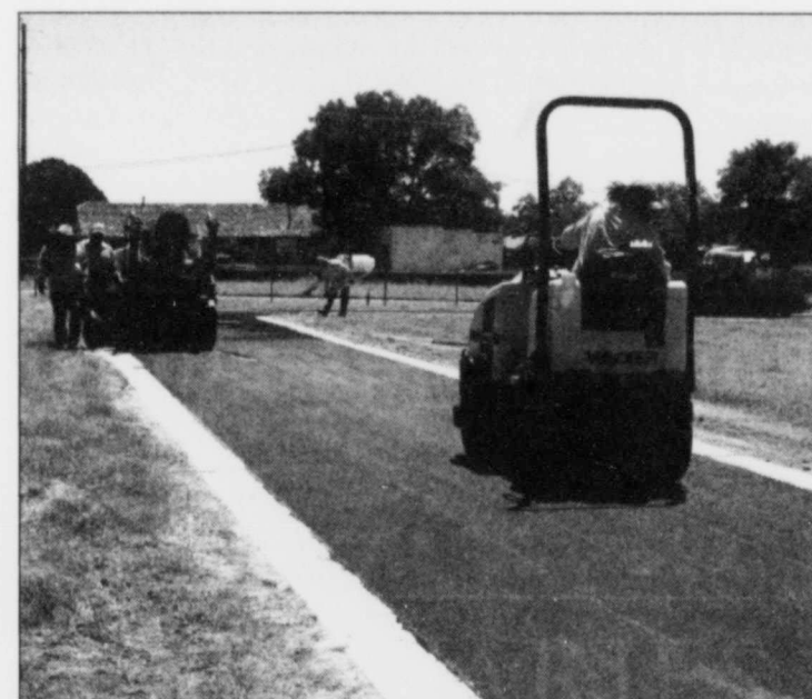
WORKERS LAY ASPHALT on the newly resurfaced track at Hutchinson Elementary. The track will be ready in time for the Relay for Life fundraiser on Friday.
