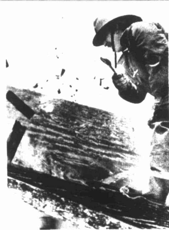
the fire under control in approximately 30 minutes. The fire started in the attic when electrical wires apparently shorted out catching some insulation on fire, according to fire department officials.
