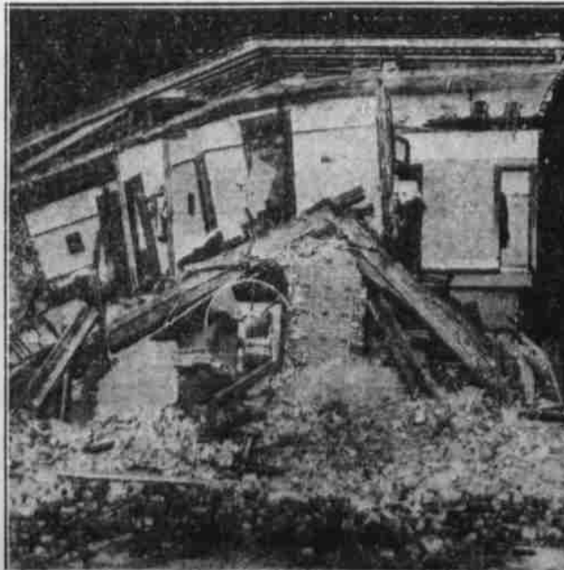
A striking example of California earthquake damage is provided by this picture of the twisted ruins of a hotel in Compton, Cal. Seven persons escaped unhurt from the structure. (Associated Press Photo)
