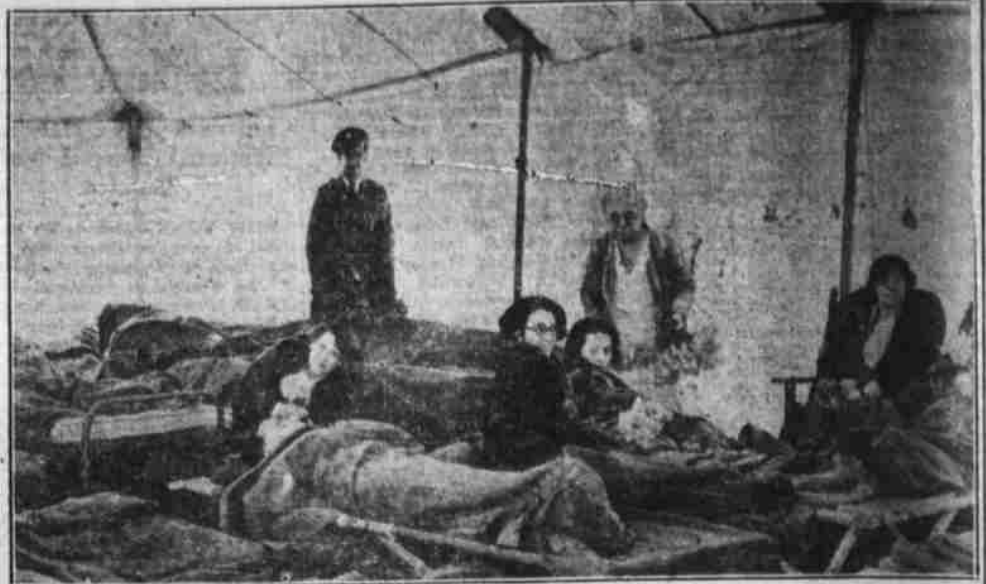
This picture provides an unusual view of emergency facilities set up to offer care to California earthquake victims. This "hospital" was organized in a tent in Long Beach to provide immediate care for the injured. (Associated Press Photo)
