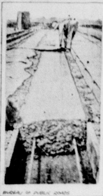
Wet burlap has been found to be the best curing treatment for concrete pavements.
