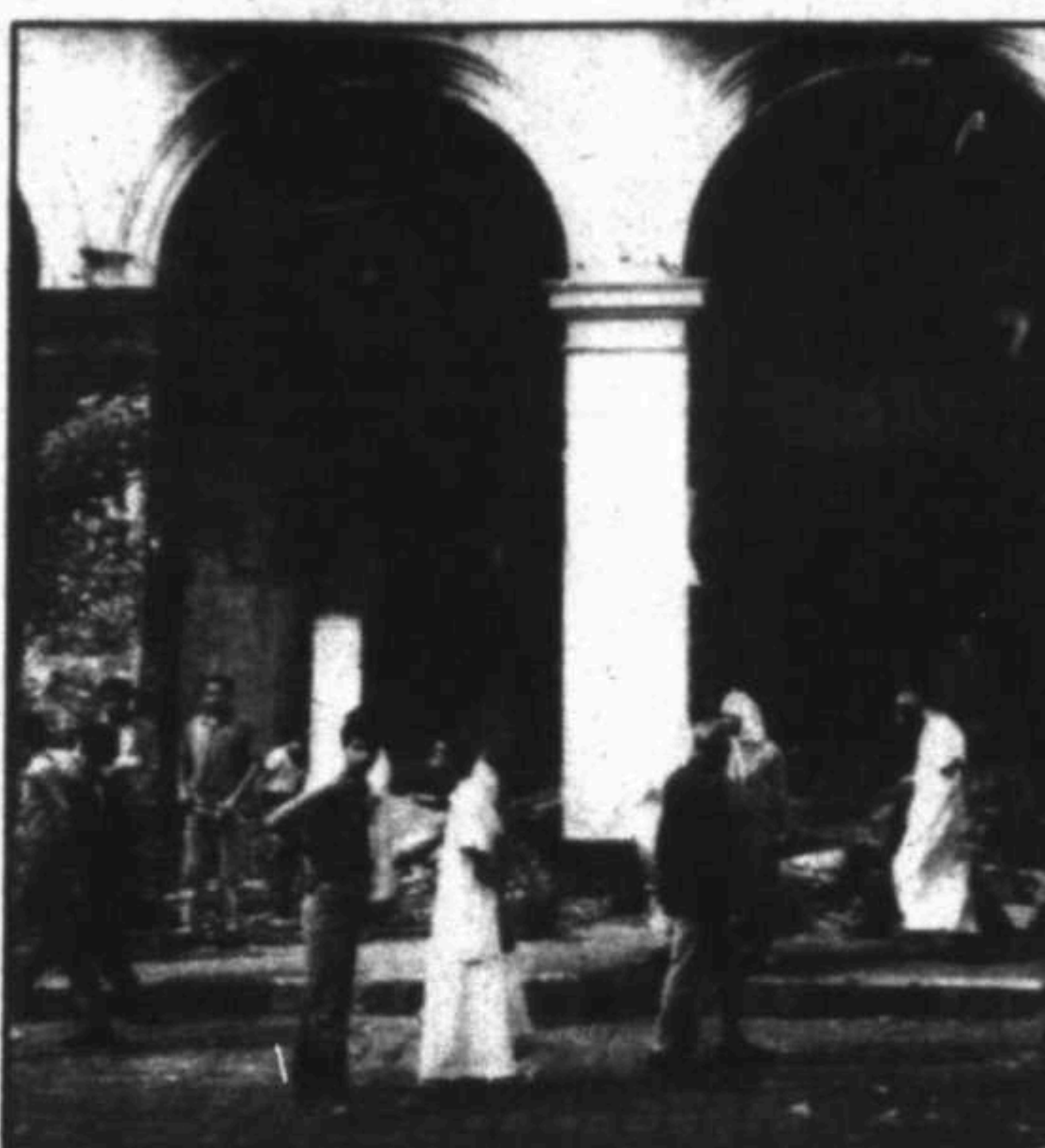
People mill in the streets of Algiers, Algeria, in front of buildings damaged by days of rioting.
