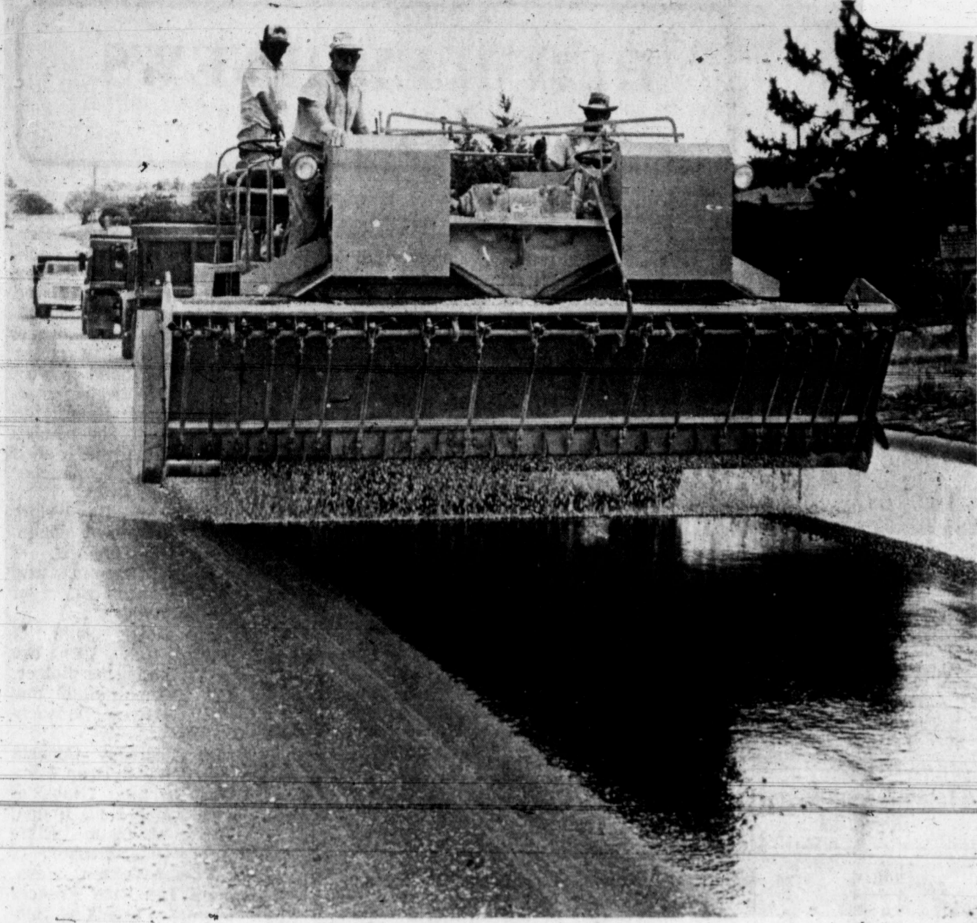
STREETS TOPPED —The annual street seal-coating program is moving along this week. Some 200 blocks of city streets are getting a new coat of asphalt and
