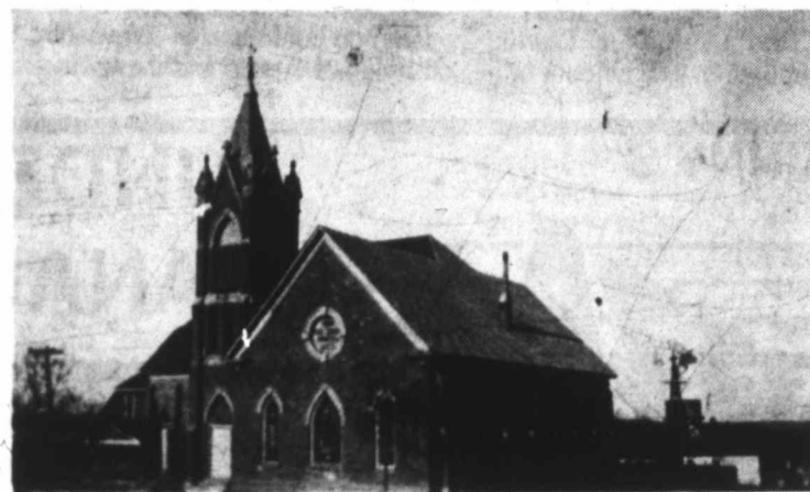
FIRST METHODIST CHURCH...constructed in 1884.
