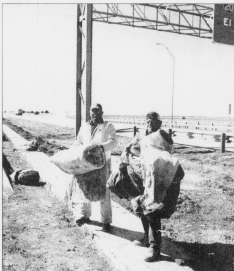
TXDOT WORKERS BEGIN laying the foundation for the construction of a median safety barrier in Mitchell County.
